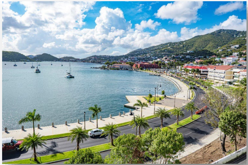
Figure 80: Phase I Veterans Drive Mitigation Improvements Project Construction Complete
