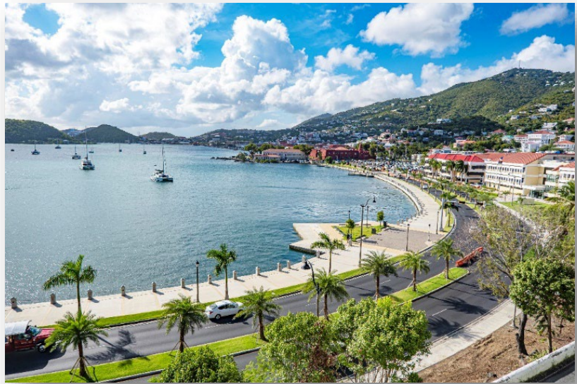
Figure 81: Phase I Veterans Drive Mitigation Improvements Project Construction Complete
