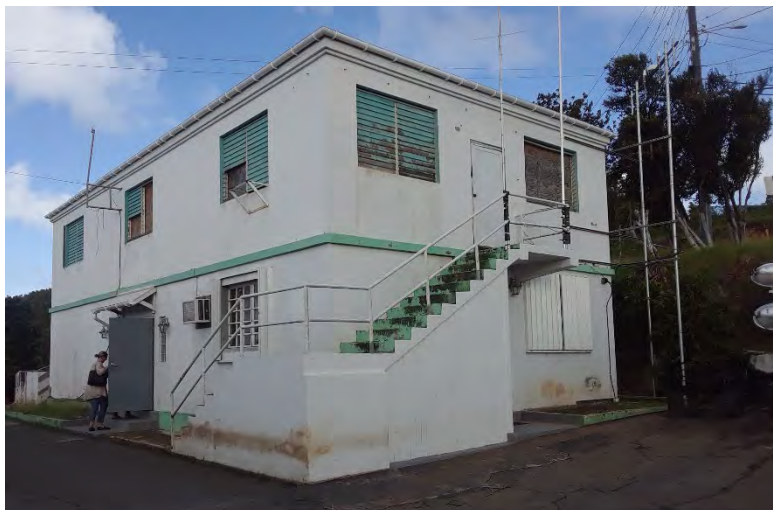
Pictured: VITEMA Emergency Operation Center on St. John.
