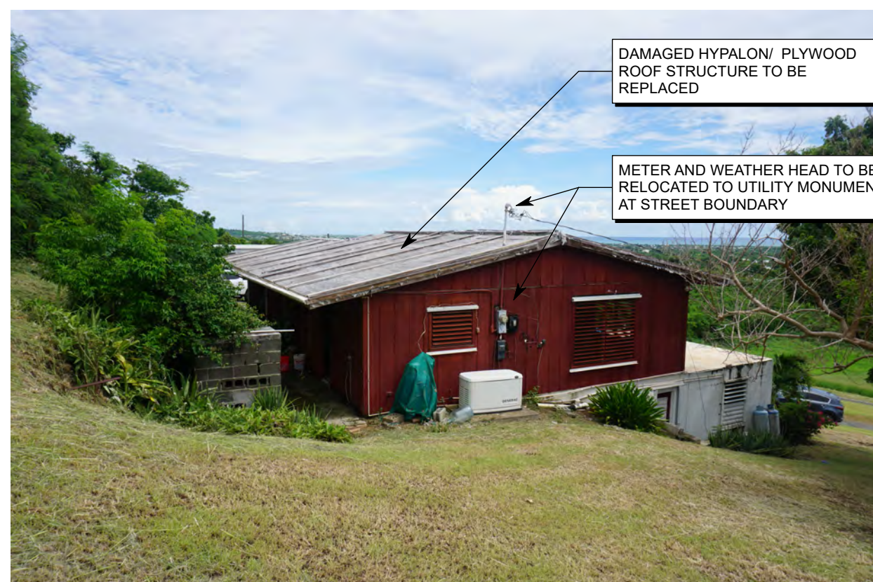
WEST VIEW: METER AND WEATHER HEAD TO BE RELOCATED TO UTILITY MONUMENT AT STREET BOUNDARY
